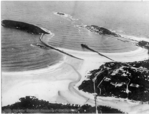
Figure 3a. Early construction of the northern breakwall in ~1926, showing Park Beach (south) and Coffs Creek mouth (Photo courtesy of the Coffs Harbour Regional Museum).
