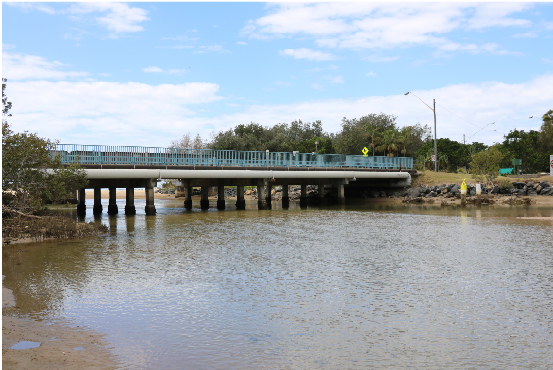
Figure 5b. The same perspective of the rail bridge with the road bridge in the foreground, Coffs Creek, 12 October 2016.
